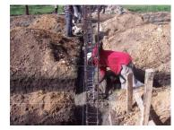
the new recommendations. The man who is in charge of this project told me there is a lot of clay in the soil, and he has planned the foundation accordingly. By this time next week, none of this work may be visible, but it will be a solid base for the rest of the building. We plan to continue as long as funds for the project are available.
